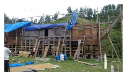
Figure 2. Installation of pole and wall construction has been completed (Banua Sikapu'mi) Source: Research Results
